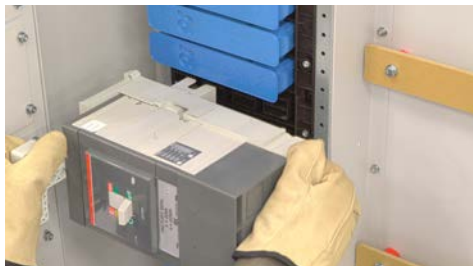
The Breaker Is Inserted Into The SafePanel
