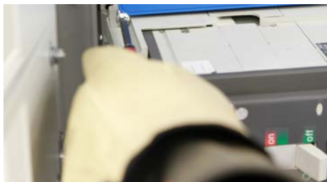
Screws Help Secure The Breaker
